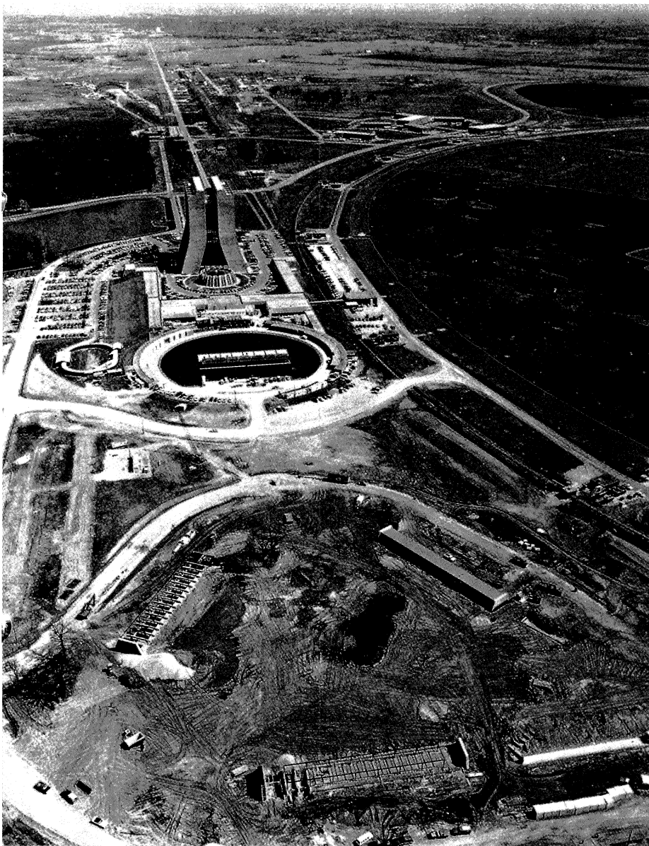
Aerial view at Fermilab, showing in the foreground the preparations for the new antiproton storage facilities. On the right is an arc of the large ring housing the conventional and superconducting magnet machines, and stretching away into the distance are the fixed target experimental areas.
